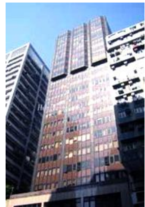
BOC Wan Chai Commercial Centre
